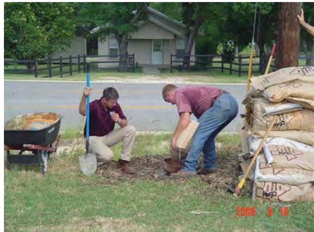
The demonstration showed the proper way to plug a drilled well and emphasized the importance of plugging abandoned wells to prevent groundwater contamination.
