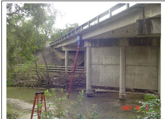
Installation of stream flow gauge at upstream site.
