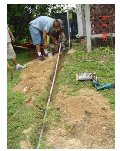
Installation of stream flow gauge at the downstream site.
