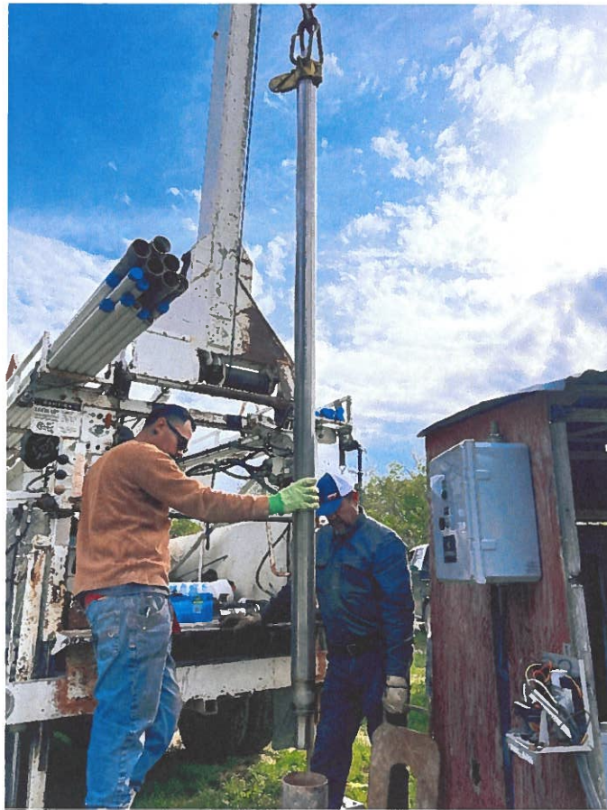
Figure 1 – MuniPak Screen Installation in Well
