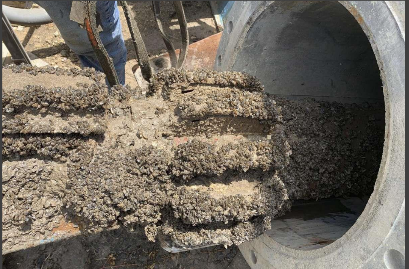
Zebra mussels encrust water intake structure
