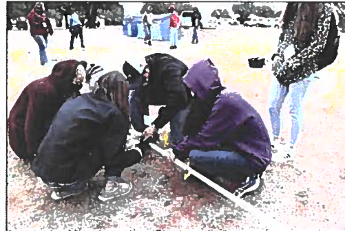
Installing the irrigation mainline
