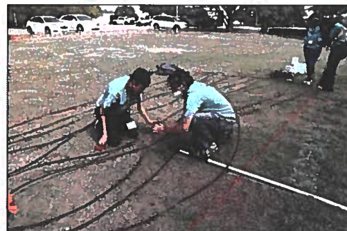
Installing drip irrigation tubing
