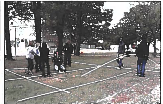
Installing lateral pipe for each station
