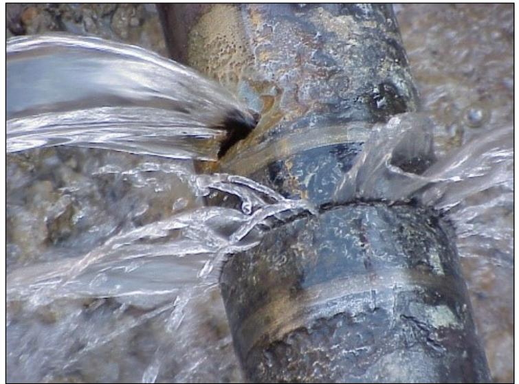
Water leaking from a supply line
