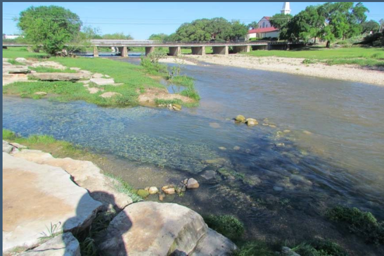
Constructed Rock Dam
