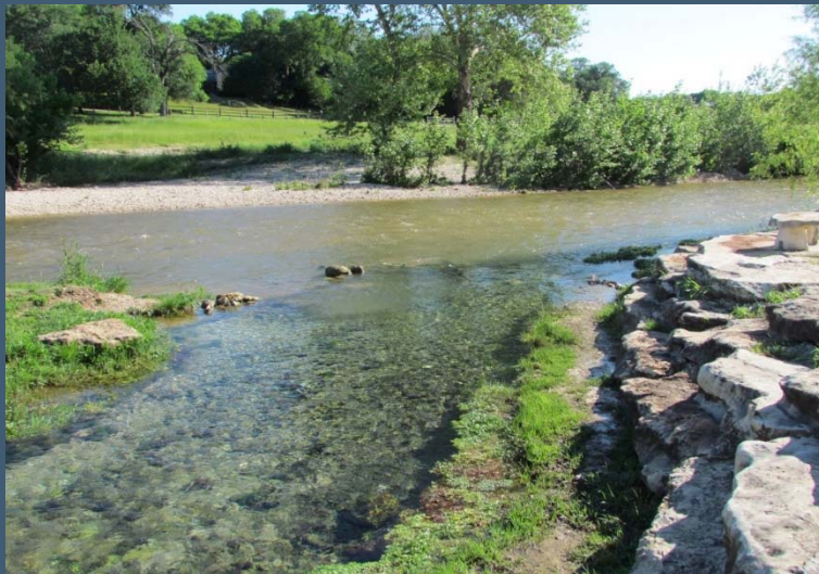
Constructed Rock Dam
