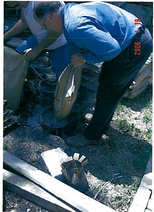
Well plugging demonstration 4-19-06
